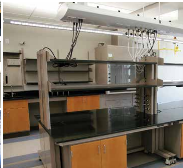
Overhead service enclosure with quick connect fittings
