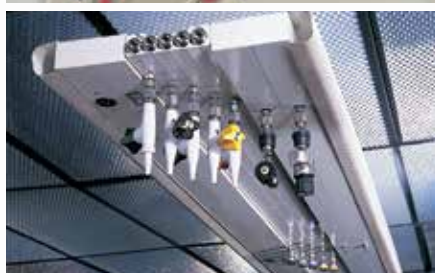
Overhead service enclosure with quick connect fittings
